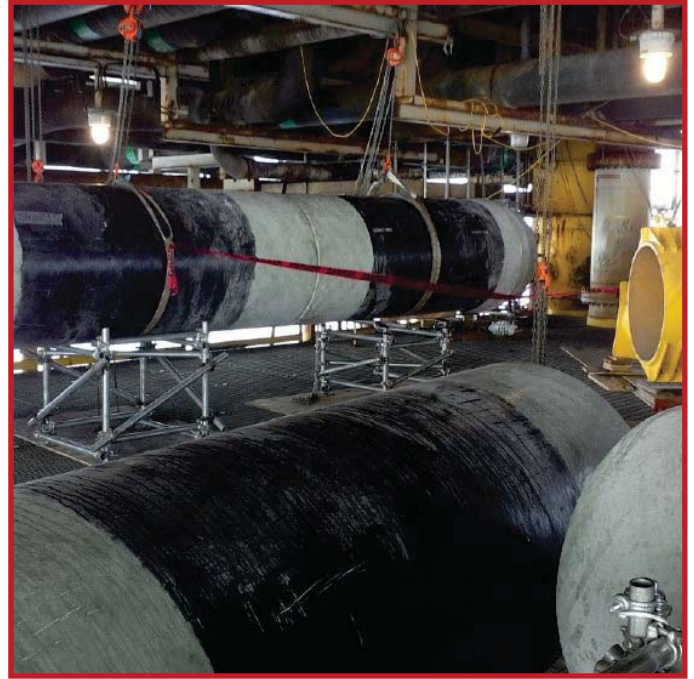
Prepping 42" Firebond and Fit up for Field Welds
