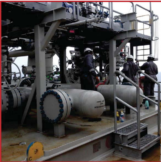
Installation of WHP Metering Skid
