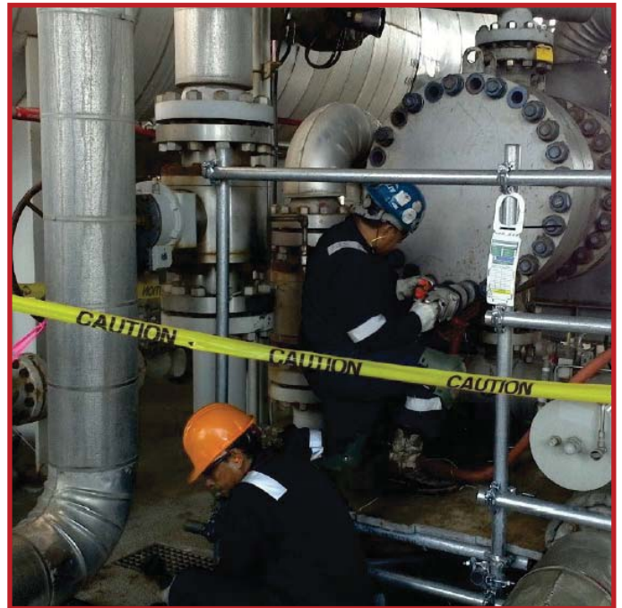
Hot Bolting Exchanger to Remove Channel Head Cover for tube Inspection
