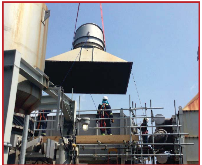
Installation of WHRU 3 (EBN-6800) Vent Stack
