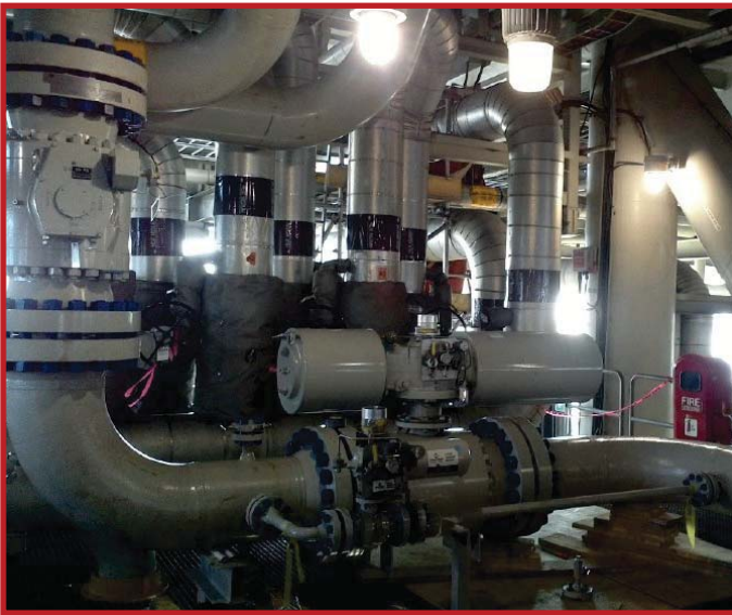
Completed Installation of 18" 2245 Spools to Section Scrubber
