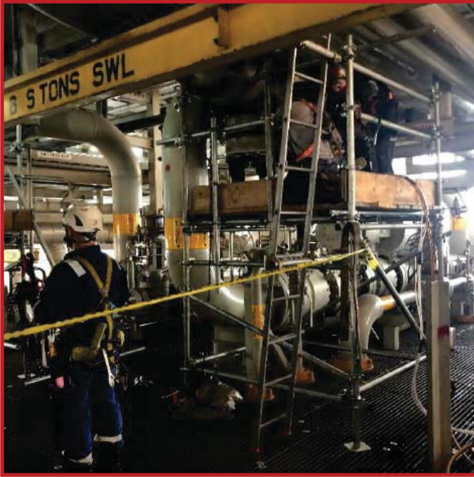
Maintenance - Strainer and Scaffolding Installation
