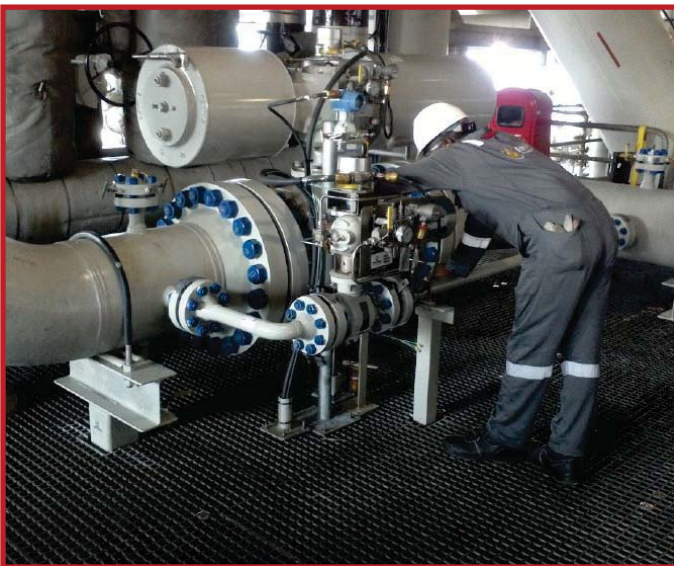
Installation of PDTs on CPP Production Mezz Deck
